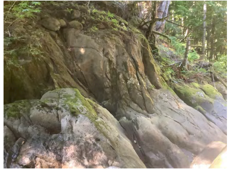
Left Bank Abutment when facing downstream
