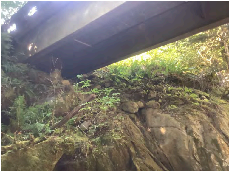
Left Bank Abutment when facing downstream
