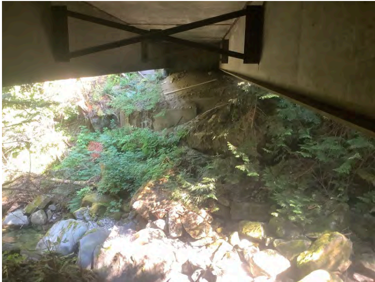
Right Bank Abutment when facing downstream
