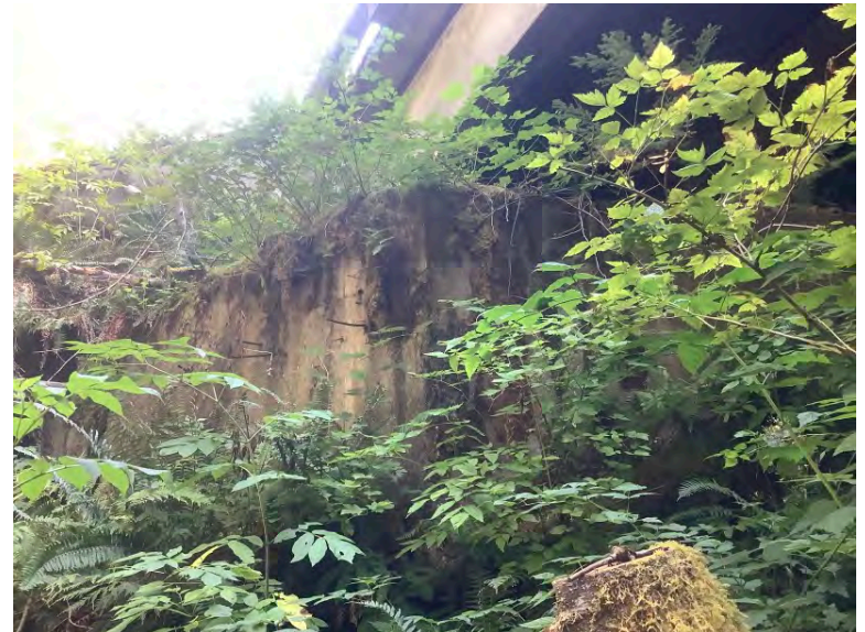
Right Bank Abutment when facing downstream
